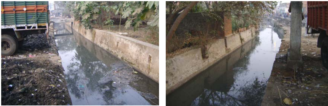
Circular Road Drain
